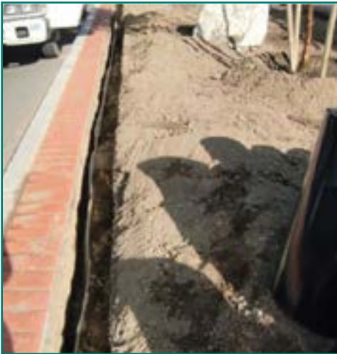
Photo Credit: SDOT Trees and Sidewalks Operations Plan
