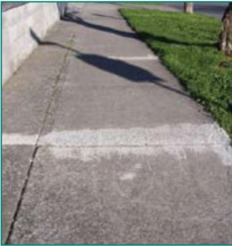
Photo Credit: SDOT Trees and Sidewalks Operations Plan
