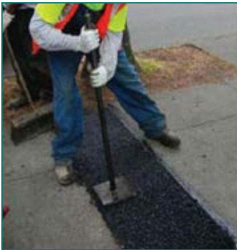
Photo Credit: SDOT Trees and Sidewalks Operations Plan
