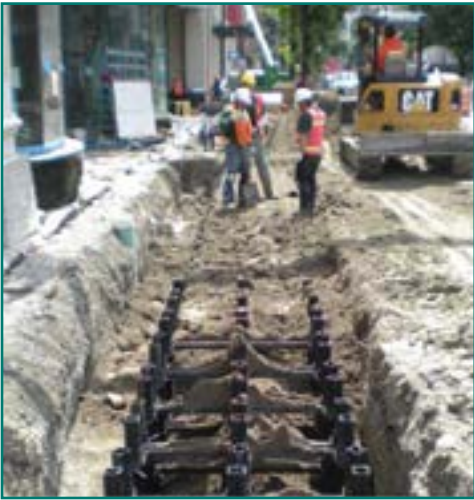
Photo Credit: SDOT Trees and Sidewalks Operations Plan
