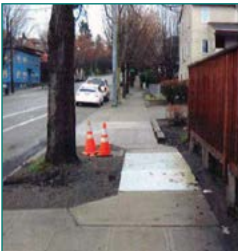
Photo Credit: SDOT Trees and Sidewalks Operations Plan
