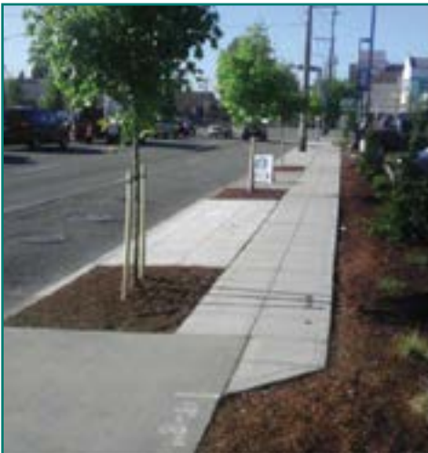
Photo Credit: SDOT Trees and Sidewalks Operations Plan
