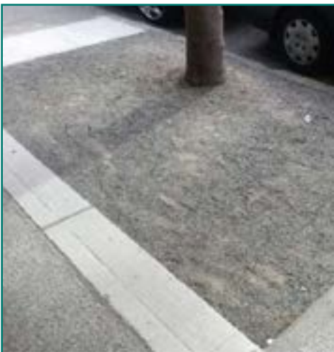
Photo Credit: SDOT Trees and Sidewalks Operations Plan
