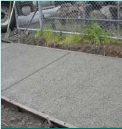
Photo Credit: SDOT Trees and Sidewalks Operations Plan
