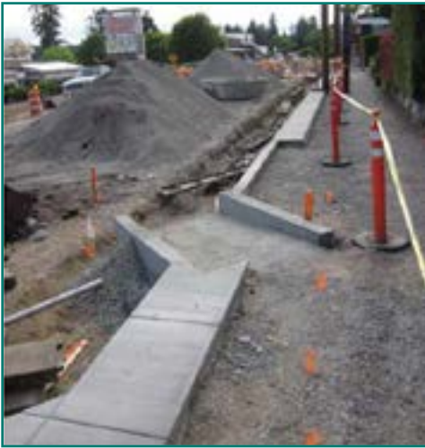
Photo Credit: SDOT Trees and Sidewalks Operations Plan
