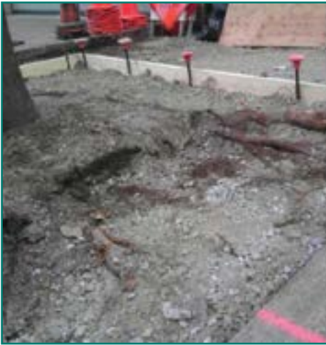
Photo Credit: SDOT Trees and Sidewalks Operations Plan
