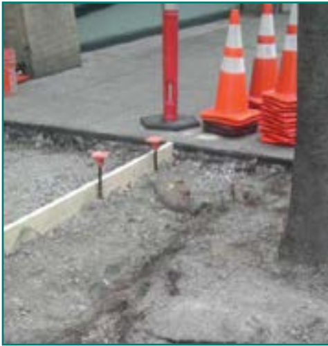
Photo Credit: SDOT Trees and Sidewalks Operations Plan
