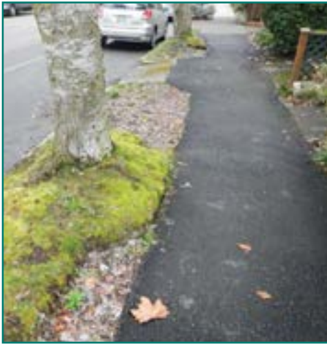
Photo Credit: SDOT Trees and Sidewalks Operations Plan
